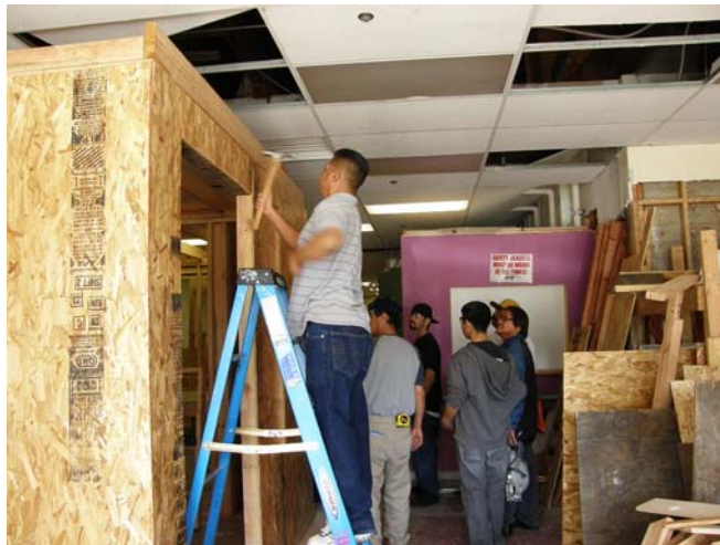
Building trainees at Centre for Employment Training develop their carpentry skills.
